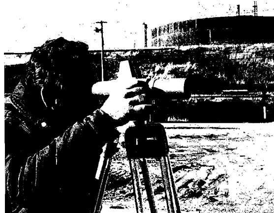
Lee Allen, project supervisor, checks grades.
