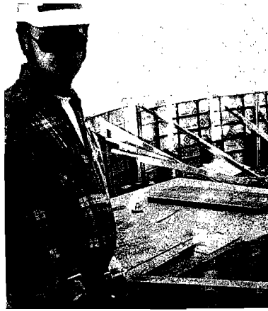
Wayne Lingo inspecting formwork.
