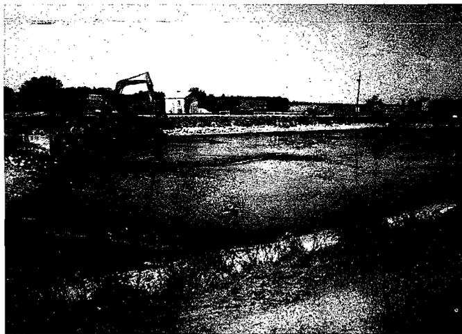
Backhoe installs new outfall line while old lagoon drains.
